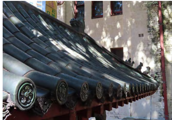
Figure 4.42 Tiles of the western side of roof.
