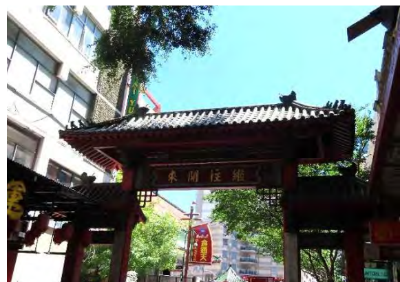
Figure 4.3 South elevation (image taken from the south).
